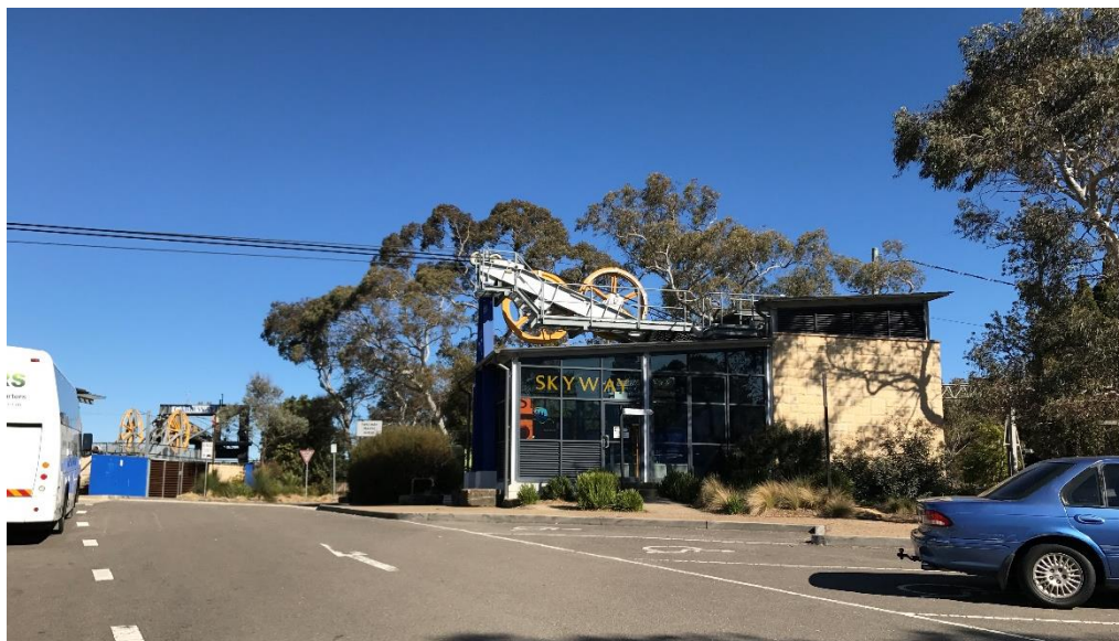
Figure 33 - View of the Skyway wheel house as seen from the parking Lot accessed from Violet Street. The KCC site is located further southwest.
