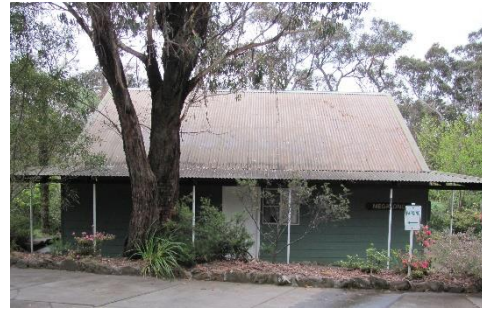
Figure 17 – Megalong located along the northern portion of the site proposed for demolition as part of the Stage 2 works.
