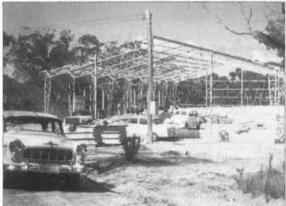
Figure 7 – Steel frame of the auditorium in 1958.
